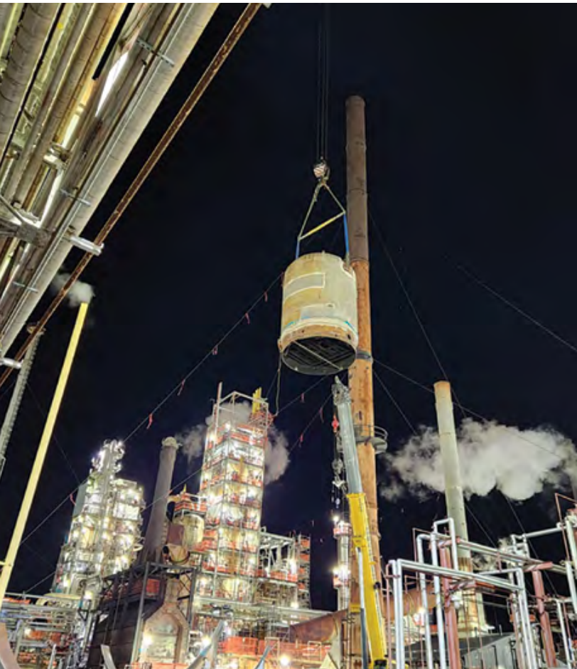
The crude top head was removed and replaced with a new overhead drum.
